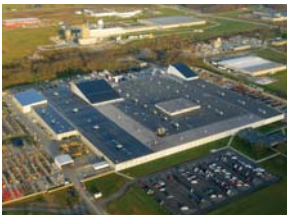
Richmond, KY - Manufacturing Plant
