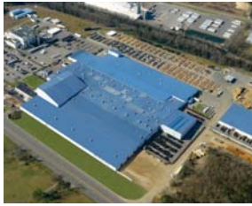
Orangeburg, SC - Manufacturing Plant
