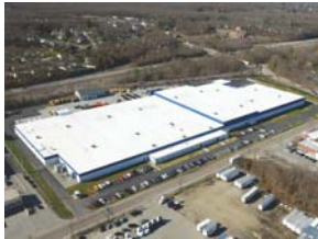
Cumberland, RI - Manufacturing Plant
