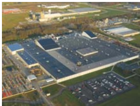
Richmond, KY - Manufacturing Plant
