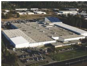
Santa Maria, CA - Manufacturing Plant
