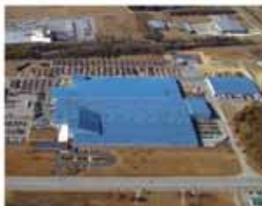
*Orangeburg, SC - Manufacturing Plant
