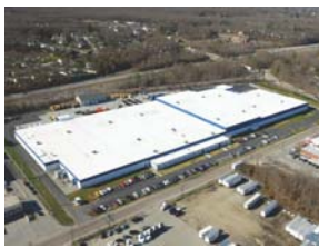
Cumberland, RI - Manufacturing Plant
