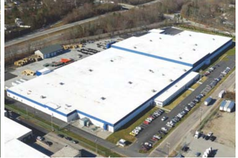
Cumberland, RI - Manufacturing Plant
