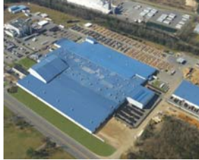
Orangeburg, SC - Manufacturing Plant
