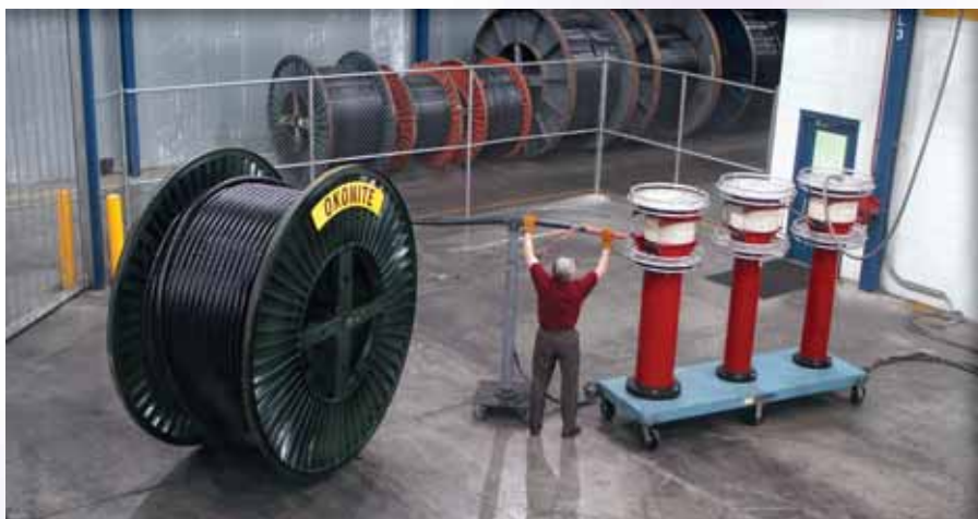
Connecting a cable to a coupling capacitor/filter for partial discharge testing.
