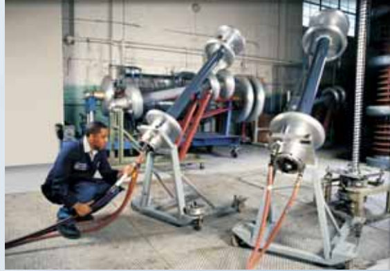
Installing an Okoguard cable into de-ionized water terminations for AC breakdown Test.
