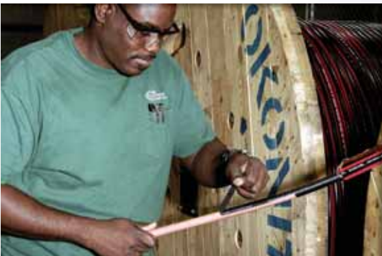
Okoguard insulated cable being terminated for test by removing the semicon layer.
