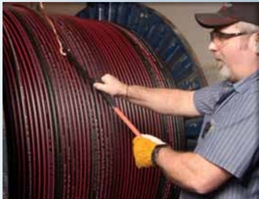
Preparing cable terminations for testing.
