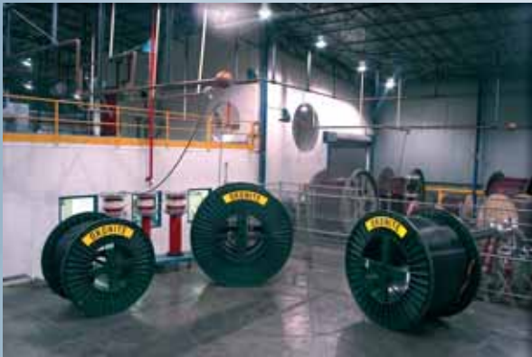
Cables awaiting partial discharge testing.
