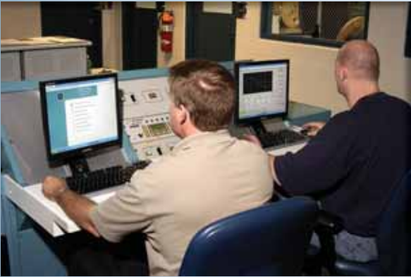
Control console for partial discharge and site location testing.
