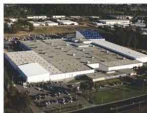
Santa Maria, CA - Manufacturing Plant
