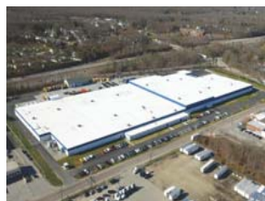
Cumberland, RI - Manufacturing Plant
