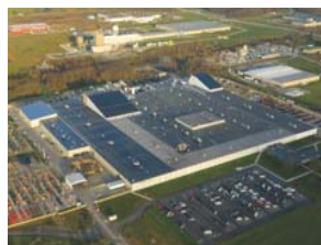
Richmond, KY - Manufacturing Plant
