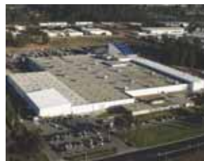
Santa Maria, CA - Manufacturing Plant
