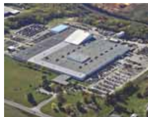
Richmond, KY - Manufacturing Plant
