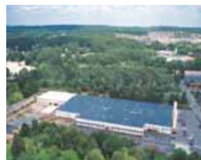
Ashton, RI - Manufacturing Plant
