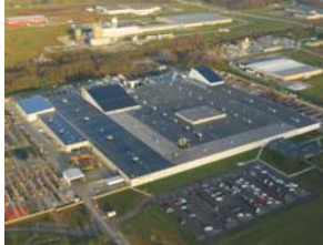
Richmond, KY - Manufacturing Plant
