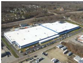
Cumberland, RI - Manufacturing Plant
