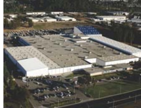
Santa Maria, CA - Manufacturing Plant
