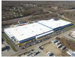
Cumberland, RI - Manufacturing Plant
