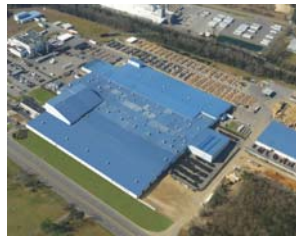
Orangeburg, SC - Manufacturing Plant
