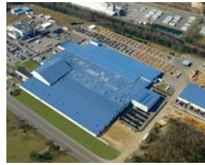
Orangeburg, SC - Manufacturing Plant
