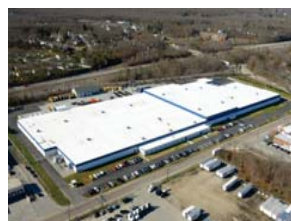
Cumberland, RI - Manufacturing Plant
