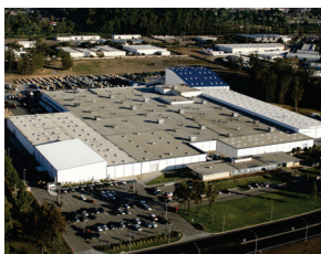
Santa Maria, CA - Manufacturing Plant
