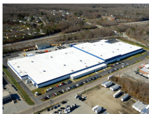
Cumberland, RI - Manufacturing Plant
