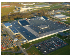
Richmond, KY - Manufacturing Plant
