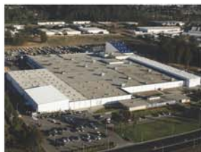
Santa Maria, CA - Manufacturing Plant
