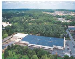
Ashton, RI - Manufacturing Plant
