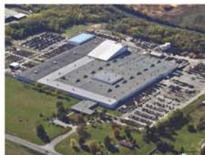
Richmond, KY - Manufacturing Plant
