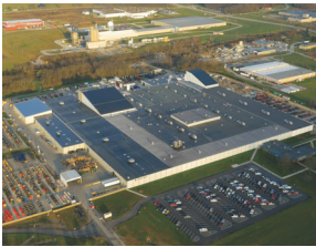
Richmond, KY - Manufacturing Plant
