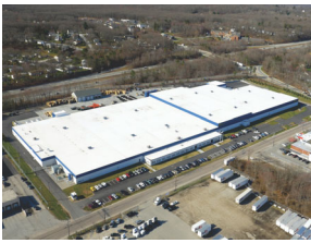
Cumberland, RI - Manufacturing Plant
