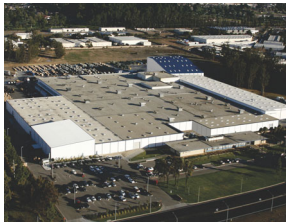
Santa Maria, CA - Manufacturing Plant
