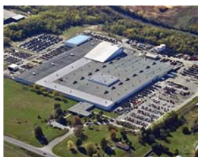
Richmond, KY - Manufacturing Plant
