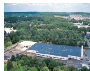
Ashton, RI - Manufacturing Plant
