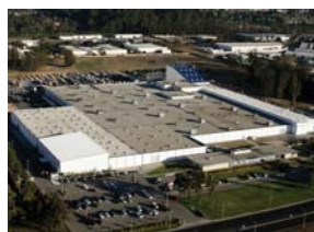
Santa Maria, CA - Manufacturing Plant
