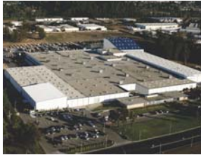
Santa Maria, CA - Manufacturing Plant
