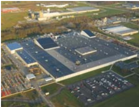
Richmond, KY - Manufacturing Plant
