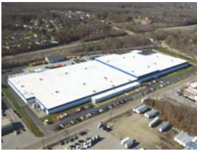
Cumberland, RI - Manufacturing Plant
