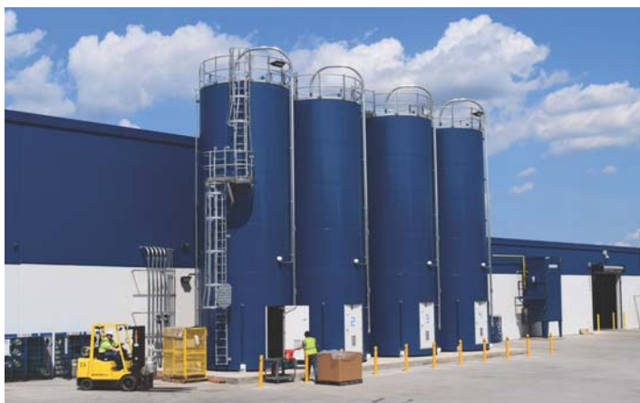
Material silos: Pelletized materials arrive in bulk and remain secure in storage.
