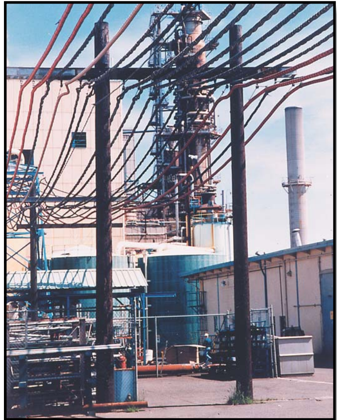
Aerial C-L-X Cable Installation
