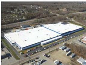
Cumberland, RI - Manufacturing Plant
