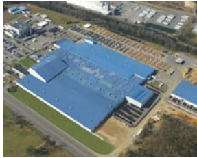
Orangeburg, SC - Manufacturing Plant
